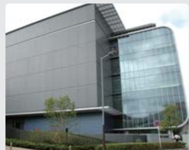
2007 Completed construction of the Yokohama Data Center 2
