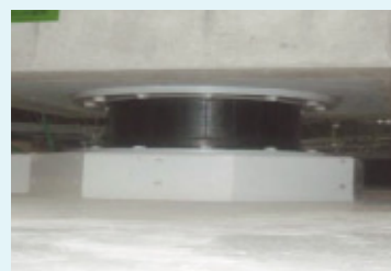
Earthquake-damage prevention through base-isolated structure
