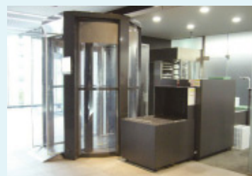
3D holographic scanners and x-ray inspection devices inspect people and items entering, exiting, and being delivered to the data center
