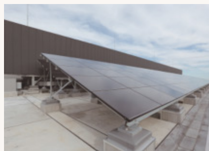
Maintenance area (rooftop: solar panels)
