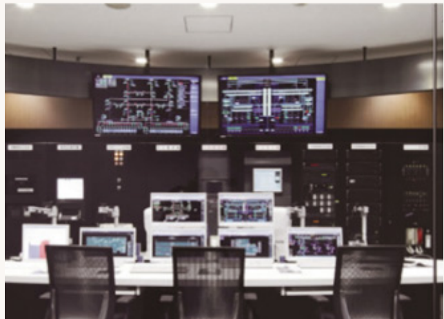
Data center central control room
