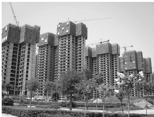
Figure 5. Condominium construction site in the suburbs of Baoji
