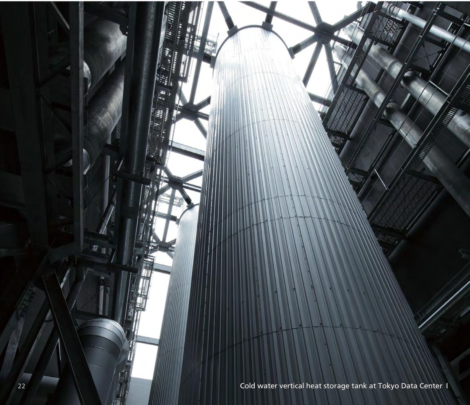
Cold water vertical heat storage tank at Tokyo Data Center I
