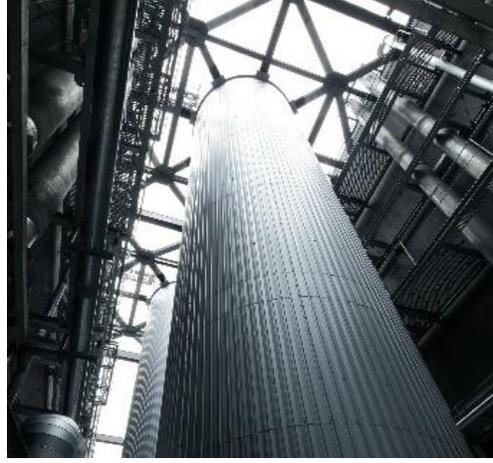
Cold water vertical heat storage tank at Tokyo Data Center 1
