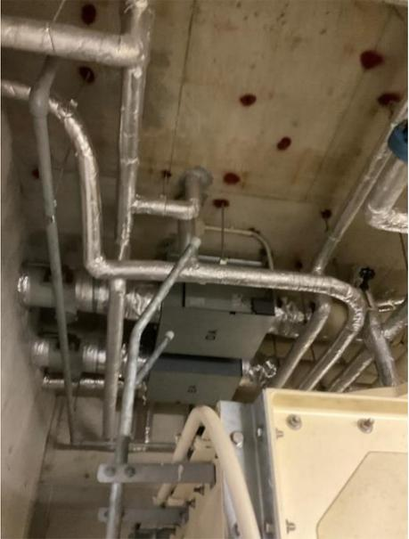
A photograph showing a complex network of pipes and machinery in a mechanical room. The pipes are wrapped in silver insulation and are connected to various pieces of equipment. | <ul style="list-style-type: none"><li>■ 場所：<br/>機械室</li><li>・ 配管用途：<br/>給水管、冷温水配管、排水管等</li></ul>       |
