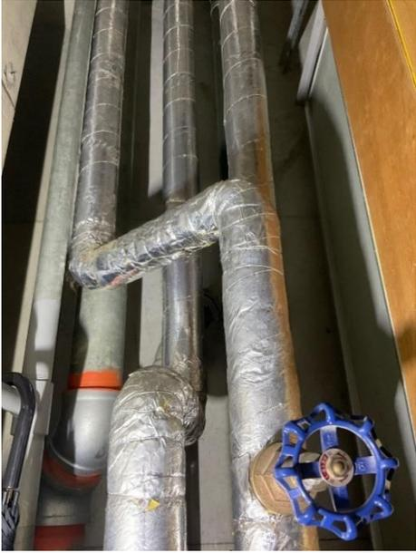
A close-up photograph of several vertical pipes wrapped in silver insulation. A blue handwheel valve is visible on the right side of the pipes.                                   | <ul style="list-style-type: none"><li>■ 場所：<br/>PS(パイプスペース)</li><li>■ 配管用途：<br/>給水管、排水管、消火管等</li></ul> |
